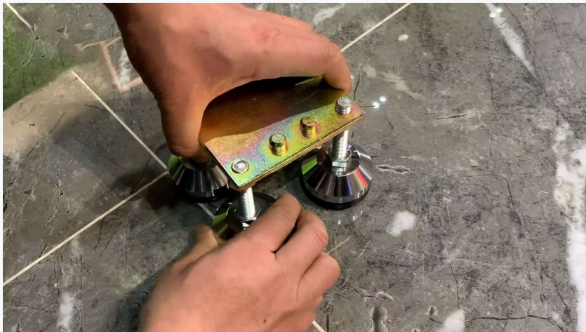
Installation of foot support
