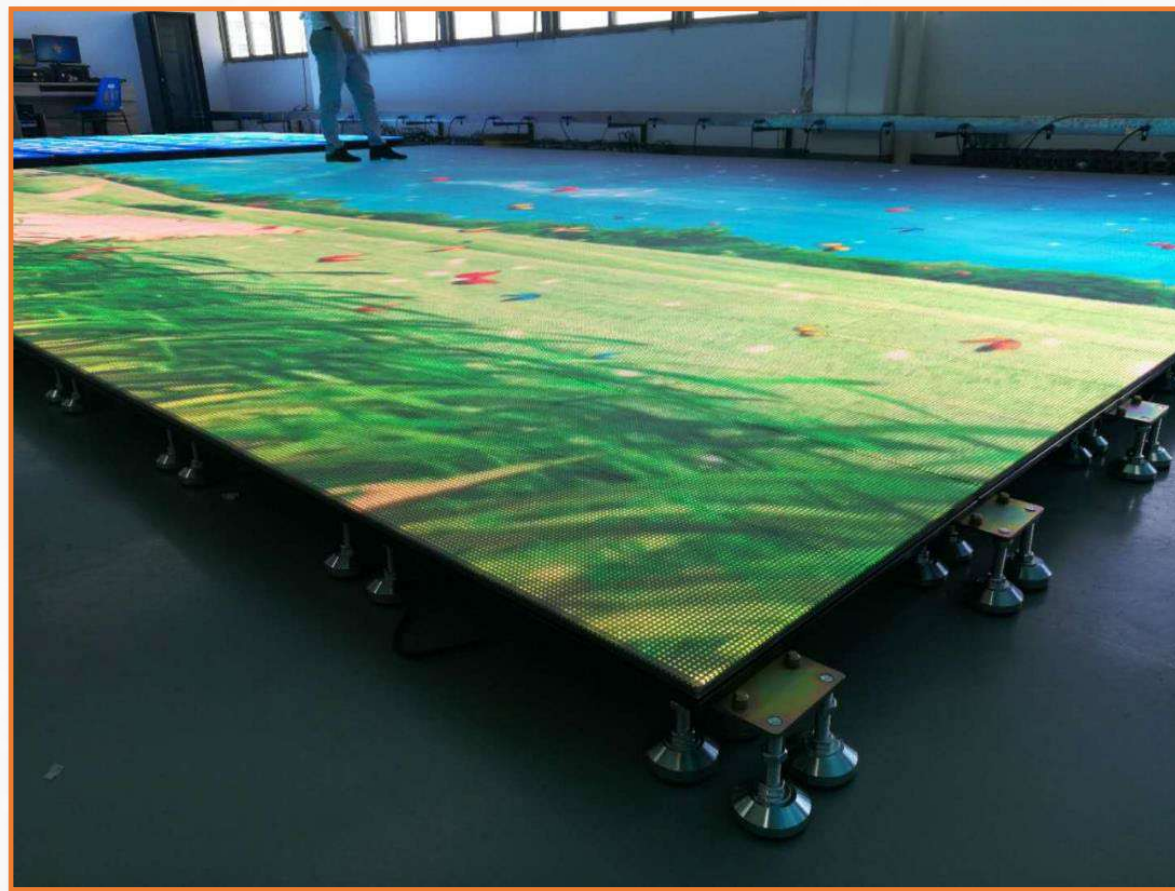
Foot stand support installation
