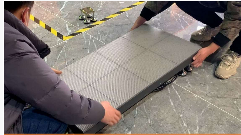
Installation of LED tile
